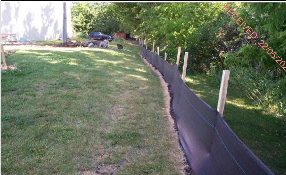
*Figure 5-21 Example of silt fence in operation on similar sites*
